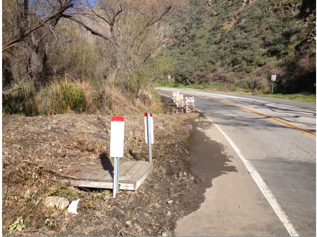
Photograph 9: North-facing view of water seepage onto Bouquet Canyon Road from the downstream end of Site 4.
