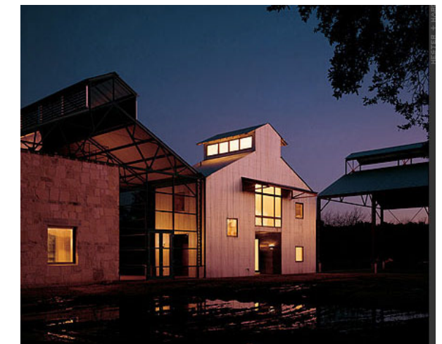
Low level light for access to parking and buildings.
